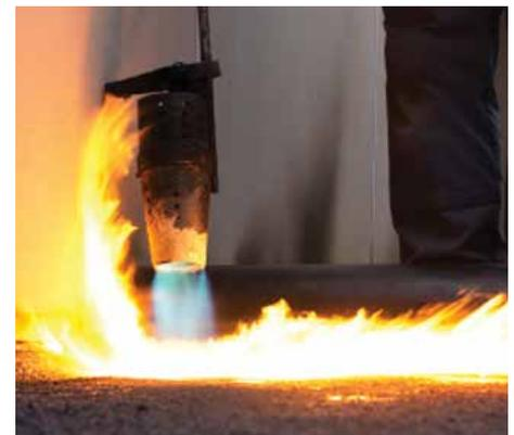
If applying a hot-melt bitumen membrane to a roof junction with a parapet wall using a flame torch, Marmox Thermoblock-PIR should be specified as this version is resistant to distortion which the standard block may experience if in contact with the flame gun. The PIR version has a slightly lower thermal conductivity (0.041W/mK), is 53mm high and like the standard version a compressive strength of 9N/mm<sup>2</sup>.
